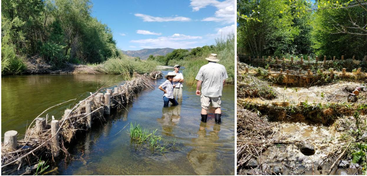
Figure 5. Photographs of various field related tasks conducted during a Beaver Dam Analogue (BDA) training hosted by the Scott River Watershed Council (SRWC) (Left: SRWC staff discussing a BDA on the Scott River; Right: BDAs constructed by the class on French Creek).
