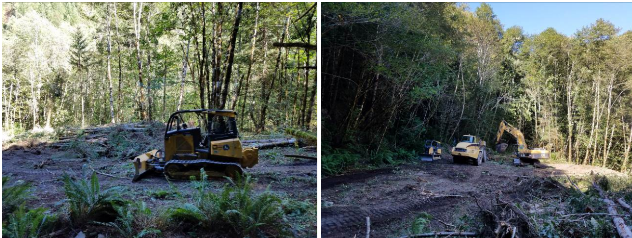
Figure 10. Photographs of road decommissioning activities in West Fork Blue Creek (09/26/17).
