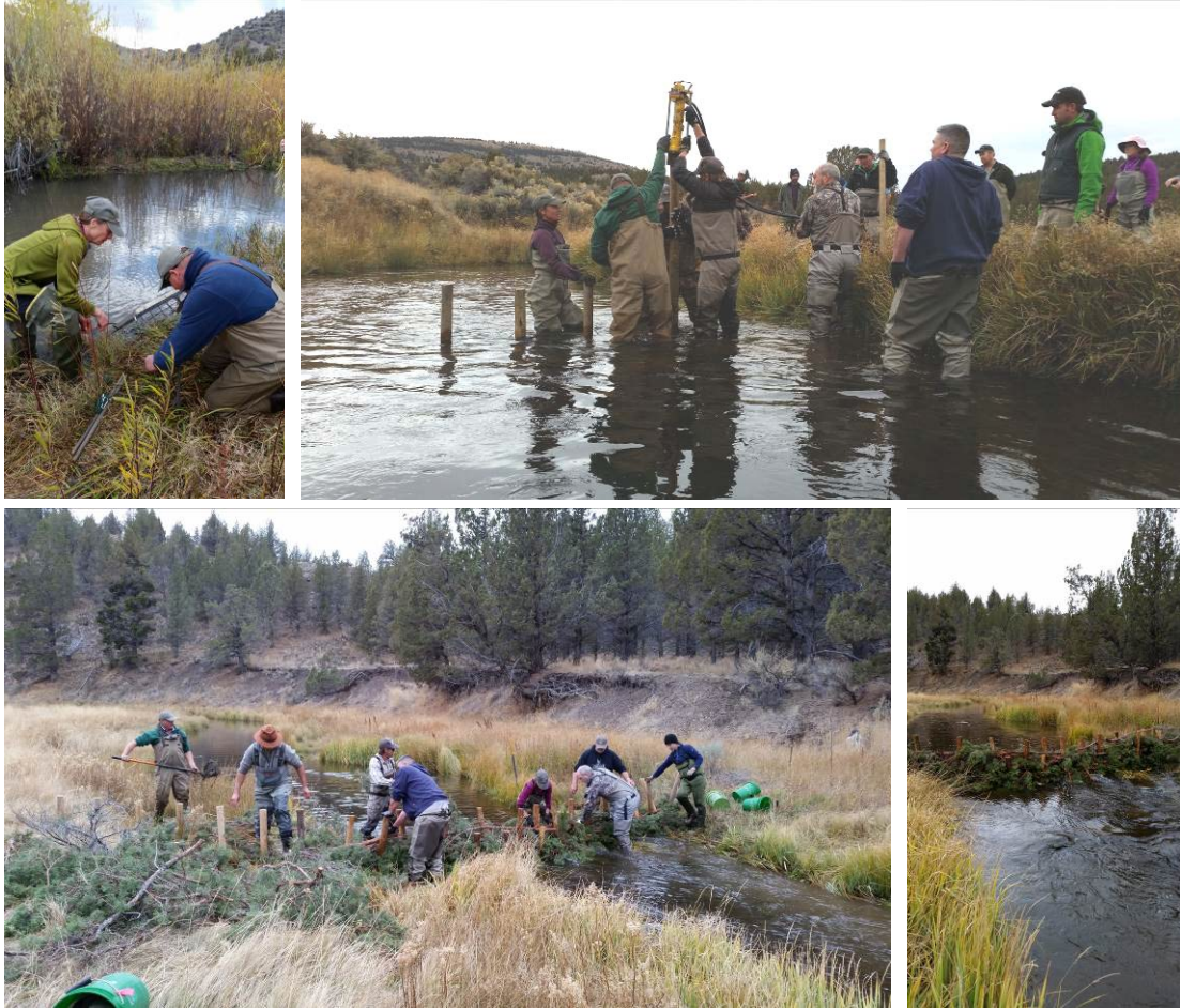
Figure 3. Photographs of various field related tasks conducted during a Working with Beaver to Restore Ecosystem Health class hosted by the Environmental Professional Program (Top Left: learning live trapping techniques; Top Right: learning to use hydraulic post pounder; Bottom Left: building a juniper limb beaver dam analogue (BDA); Bottom Right: completed BDA).
