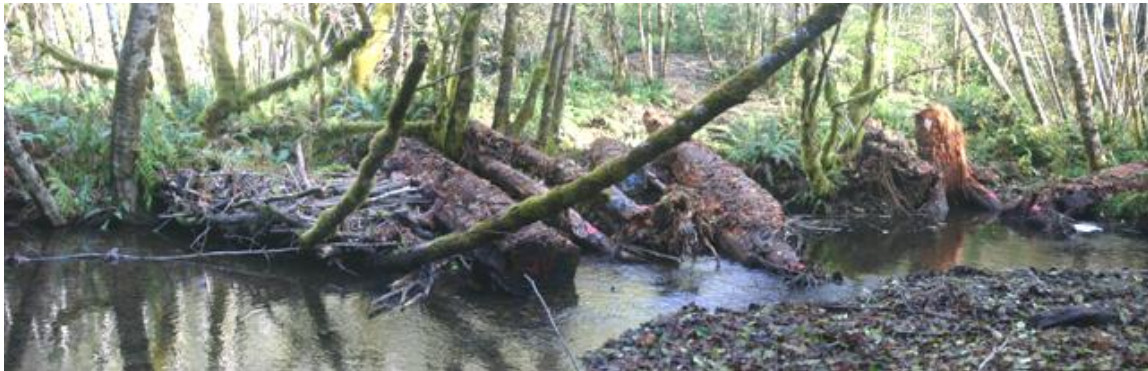
Figure 58. Confluence pool in upper portion of reach following installation of structure #6, Mainstem McGarvey Creek, Lower Klamath River, California, October 2008.
