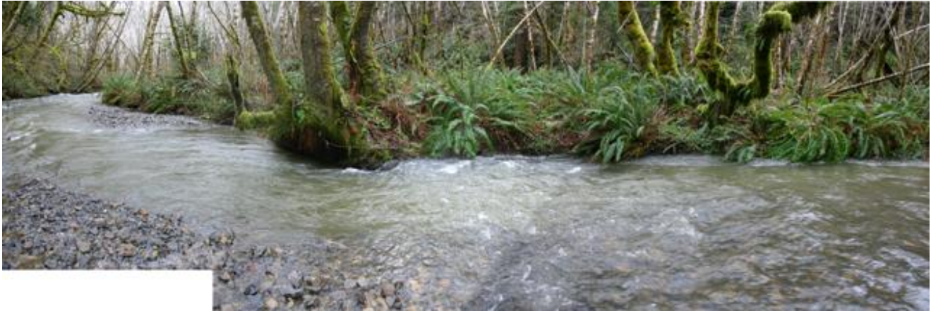
Figure 66. Lateral scour pool in middle portion of reach prior to installation of structures #8-9, Mainstem McGarvey Creek, Lower Klamath River, California, February 2007.
