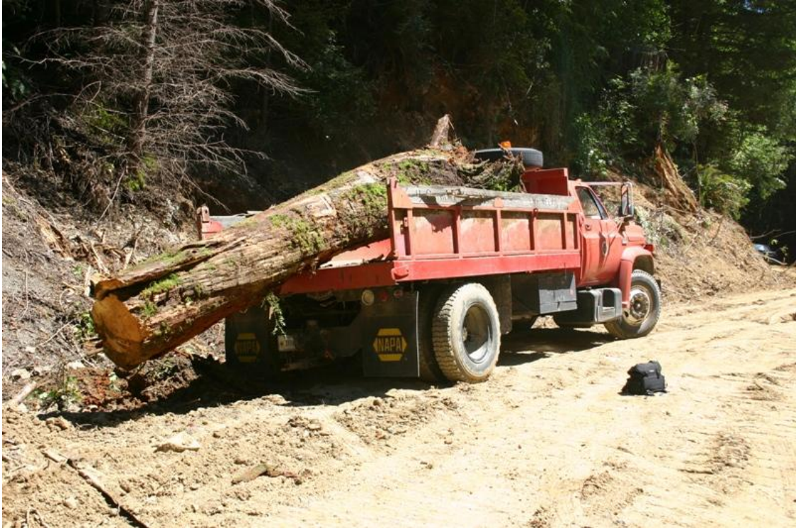
Figure 9. LWD being transported from road decommissioning site to the stockpile area, McGarvey Creek, Lower Klamath River, 2006.
