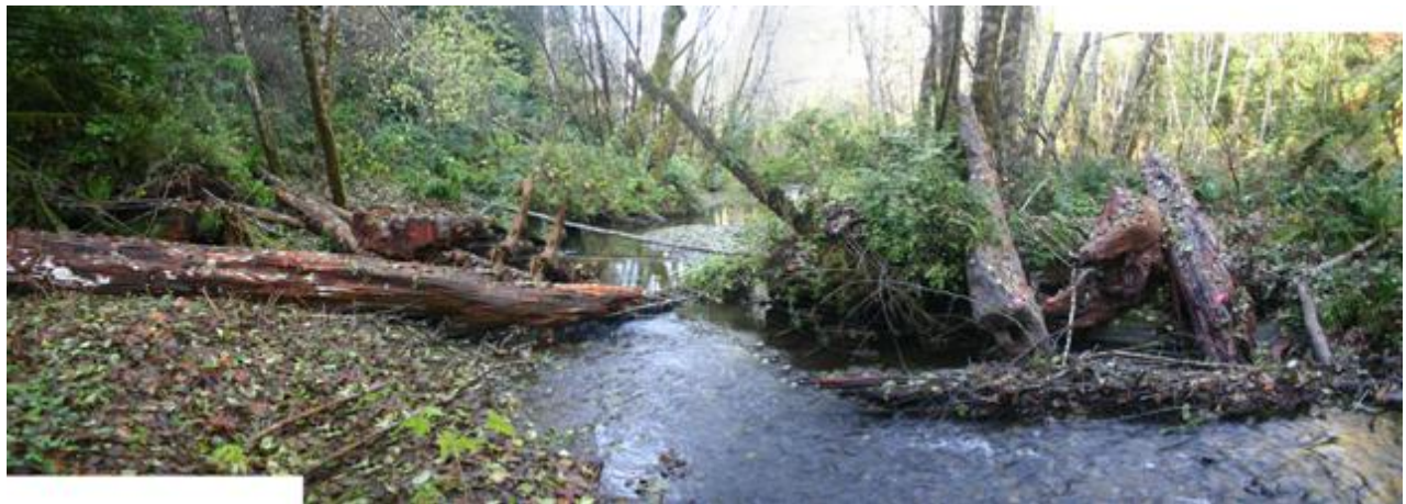
Figure 67. Scour pool in middle portion of reach following installation of structures #8-9, Mainstem McGarvey Creek, Lower Klamath River, California, November 2008.
