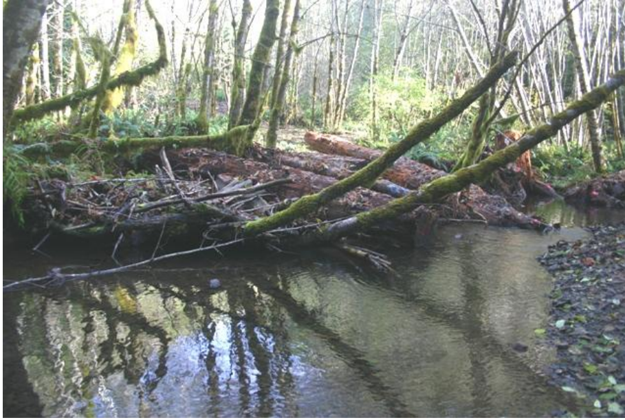
Figure 57. Confluence pool in upper portion of reach following installation of structure #6, Mainstem McGarvey Creek, Lower Klamath River, California, October 2008.
