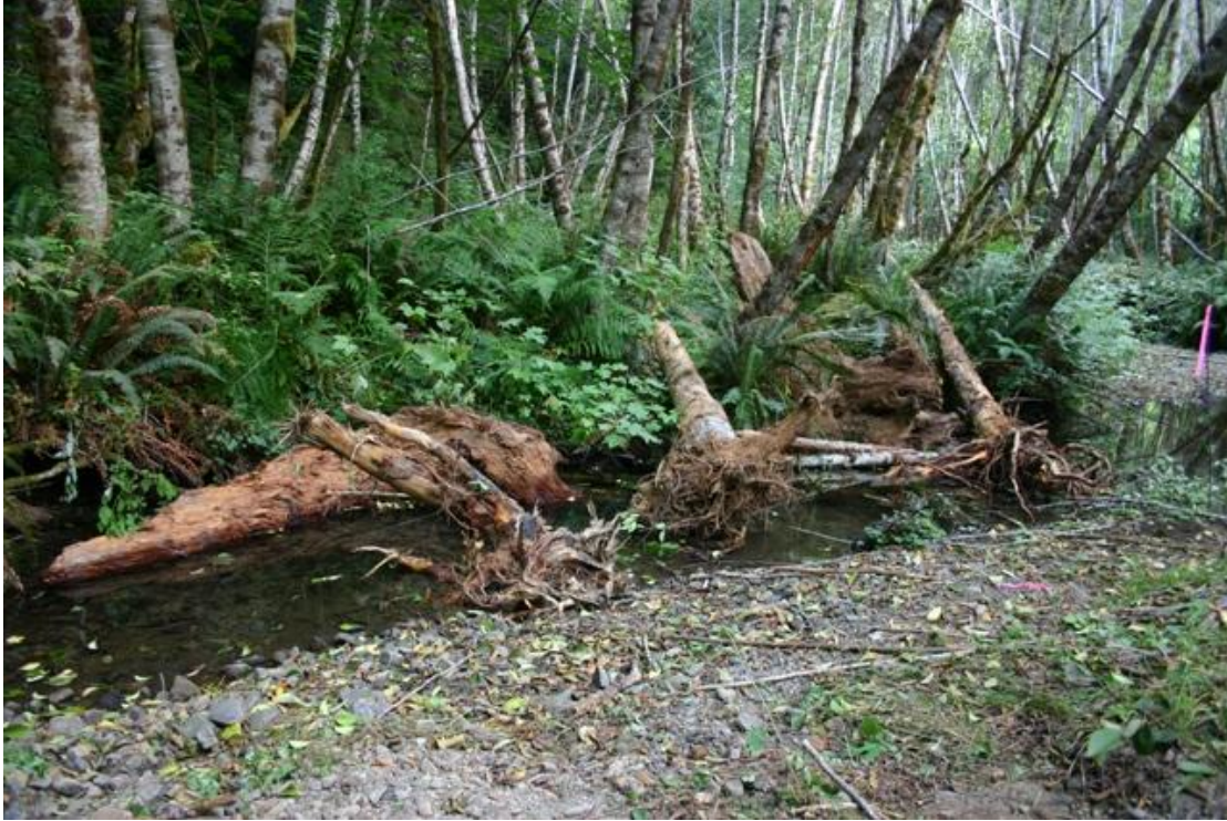
Figure 33. Shallow pool near top of project reach following installation of structure #4, Mainstem McGarvey Creek, Lower Klamath River, California, September 2008.
