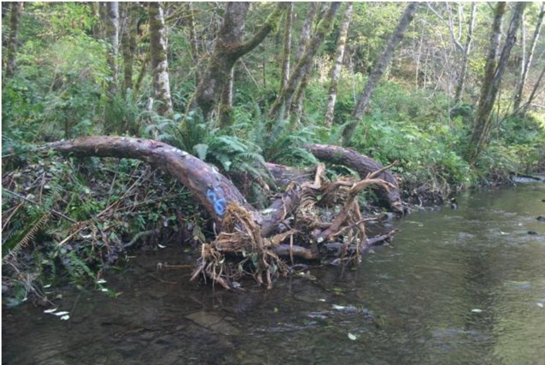
Figure 16. Shallow run at top of project reach following installation of structures #1, Mainstem McGarvey Creek, Lower Klamath River, California, September 2008.
