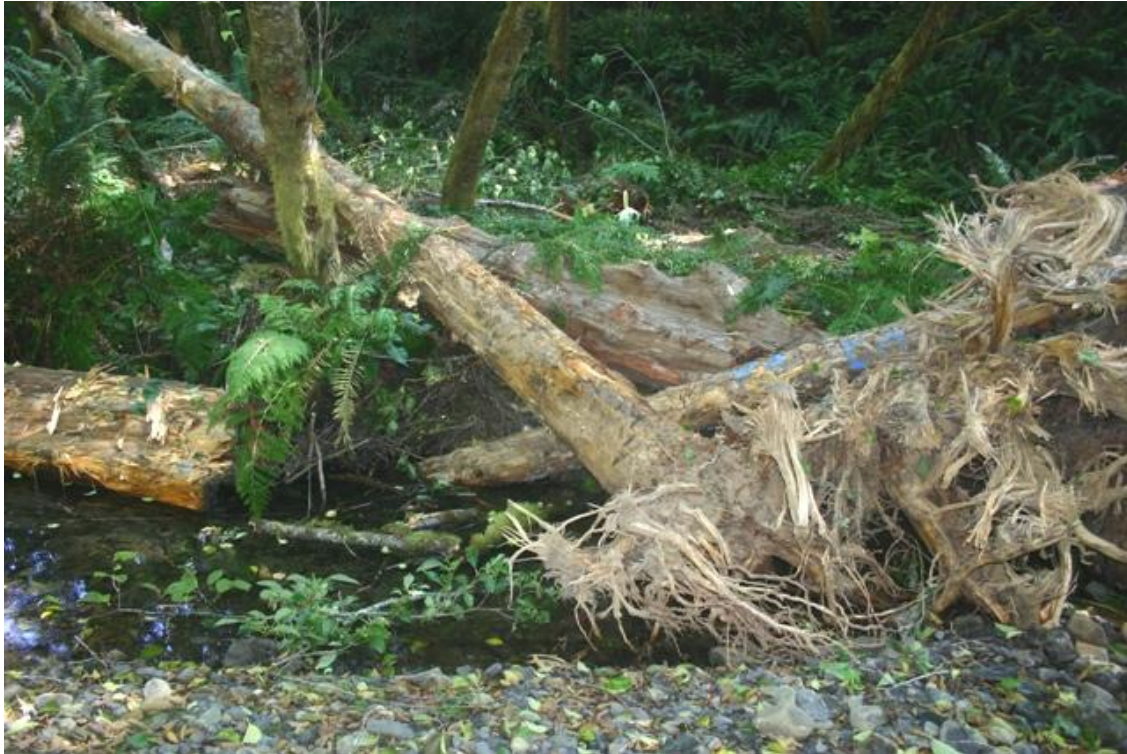
Figure 46. Shallow pool in upper portion of reach following installation of structure #5, Mainstem McGarvey Creek, Lower Klamath River, California, September 2008.
