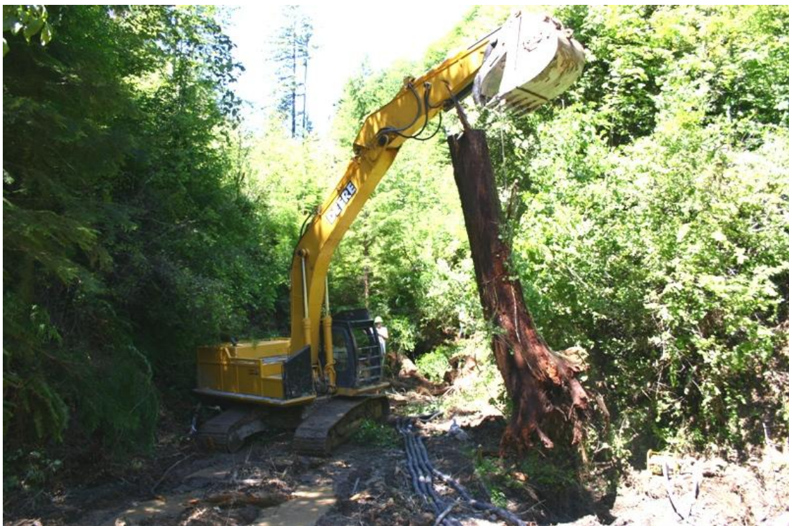
Figure 8. Large woody debris retrieved from “Humboldt” stream crossing during road decommissioning, McGarvey Creek, Lower Klamath River, California 2006.
