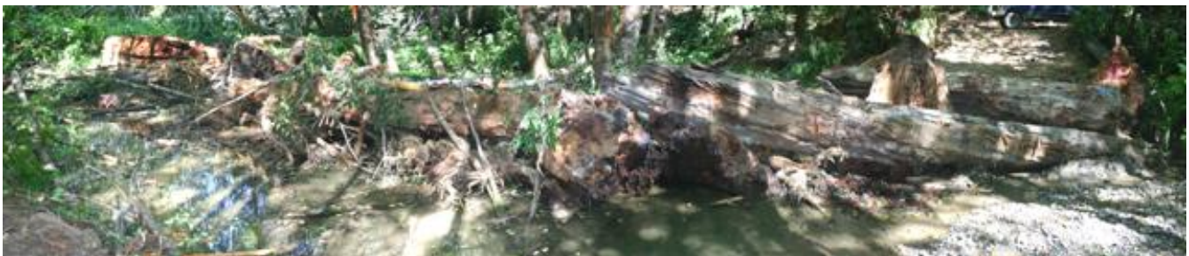
Figure 72. Step-run in middle portion of reach following installation of structures #10, Mainstem McGarvey Creek, Lower Klamath River, California, September 2008.
