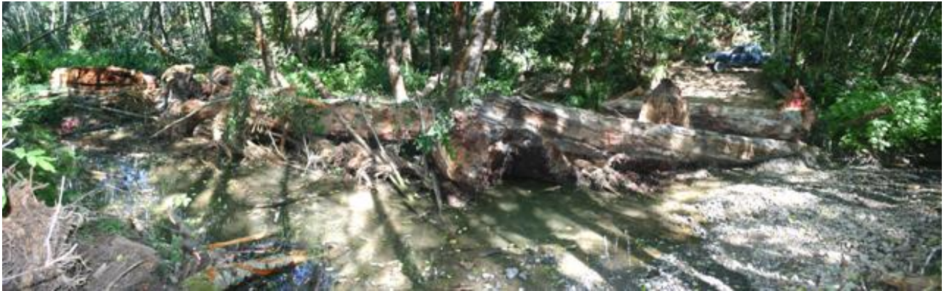
Figure 71. Step-run in middle portion of reach following installation of structures #10, Mainstem McGarvey Creek, Lower Klamath River, California, September 2008.
