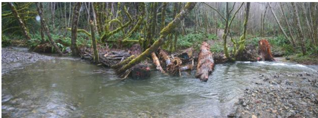
Figure 59. Structure #6 following high winter flows, Mainstem McGarvey Creek, Lower Klamath River, California, January 2009.
