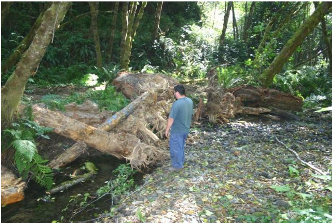
Figure 47. Shallow pool in upper portion of reach following installation of structure #5, Mainstem McGarvey Creek, Lower Klamath River, California, September 2008.
