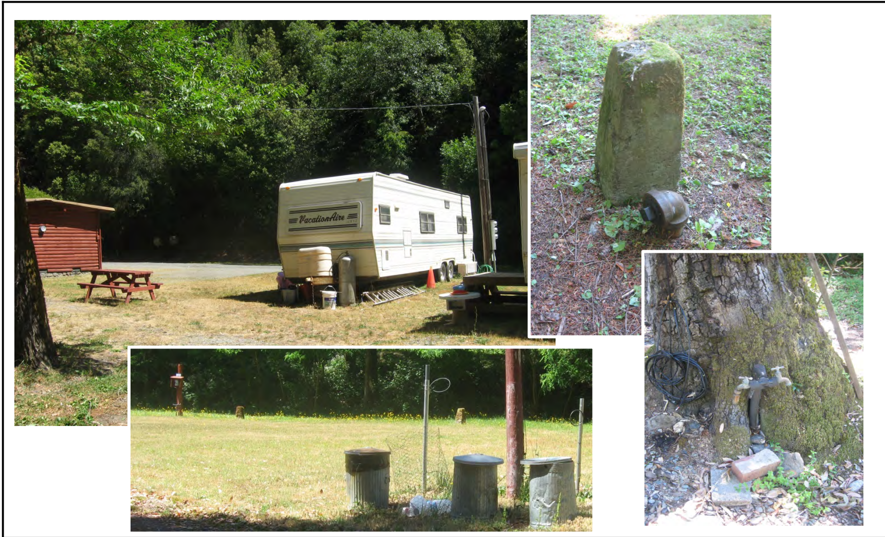
Upper Right: Standard RV site with shower/toilet outbuilding visible to left. Lower Right: Trash cans and wire container for recyclable cans and bottles; electrical connection pole in distant left. Upper left: Septic connection and protective concrete monument.. Lower Left: Water supply
