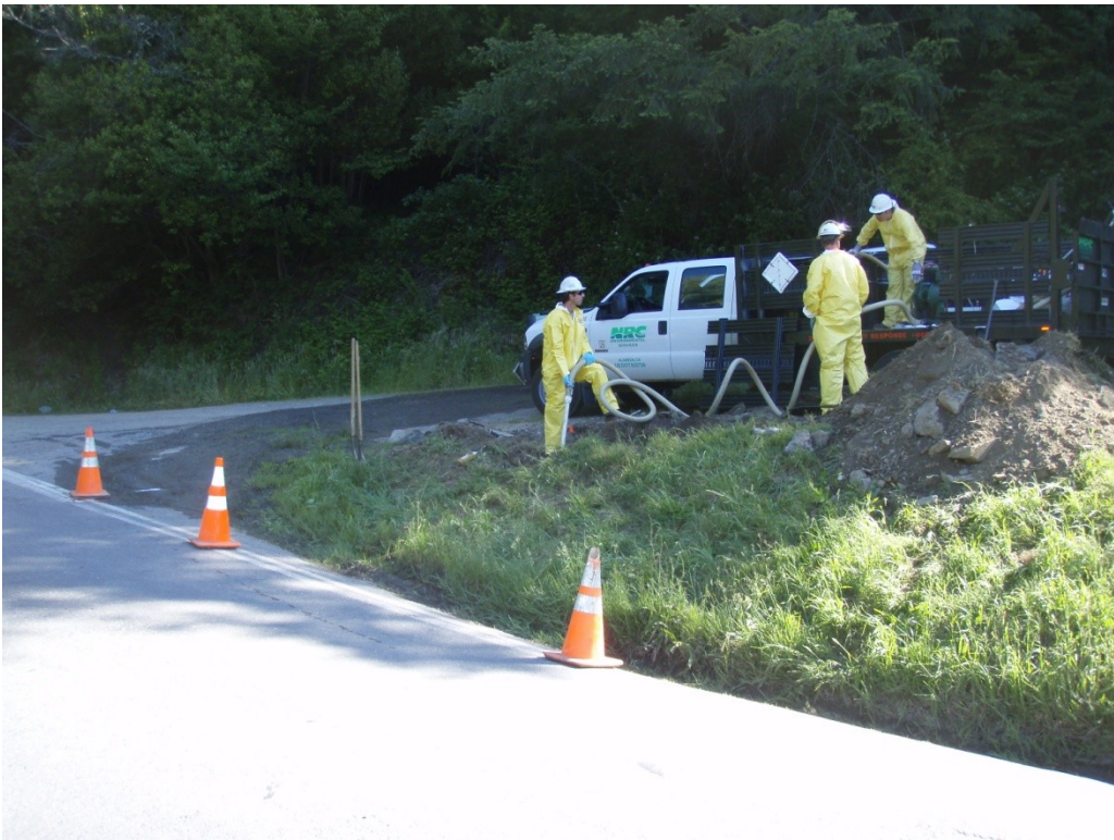
Photo 04: Removing contents of the UST. Followed by triple rinsing and final pumping. Direction: North
