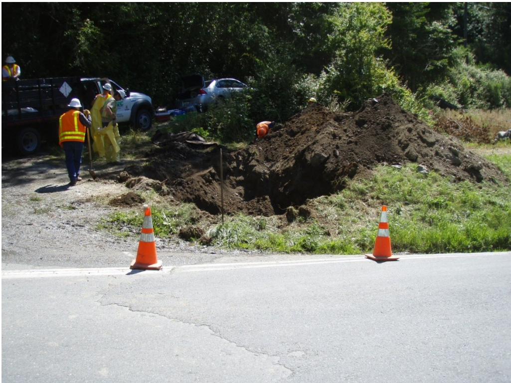
Photo 06: UST excavation after UST removal and prior to backfilling. Direction: Northeast
