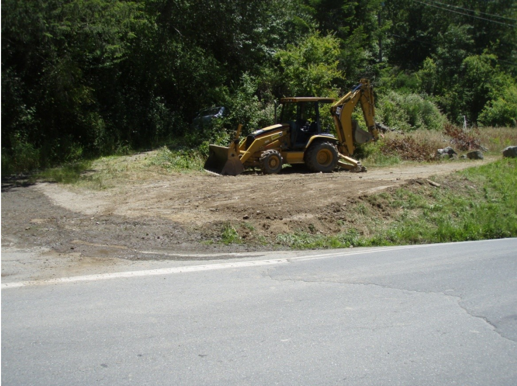
Photo 08: Site following assessment activities and final grading. Direction: Northeast
